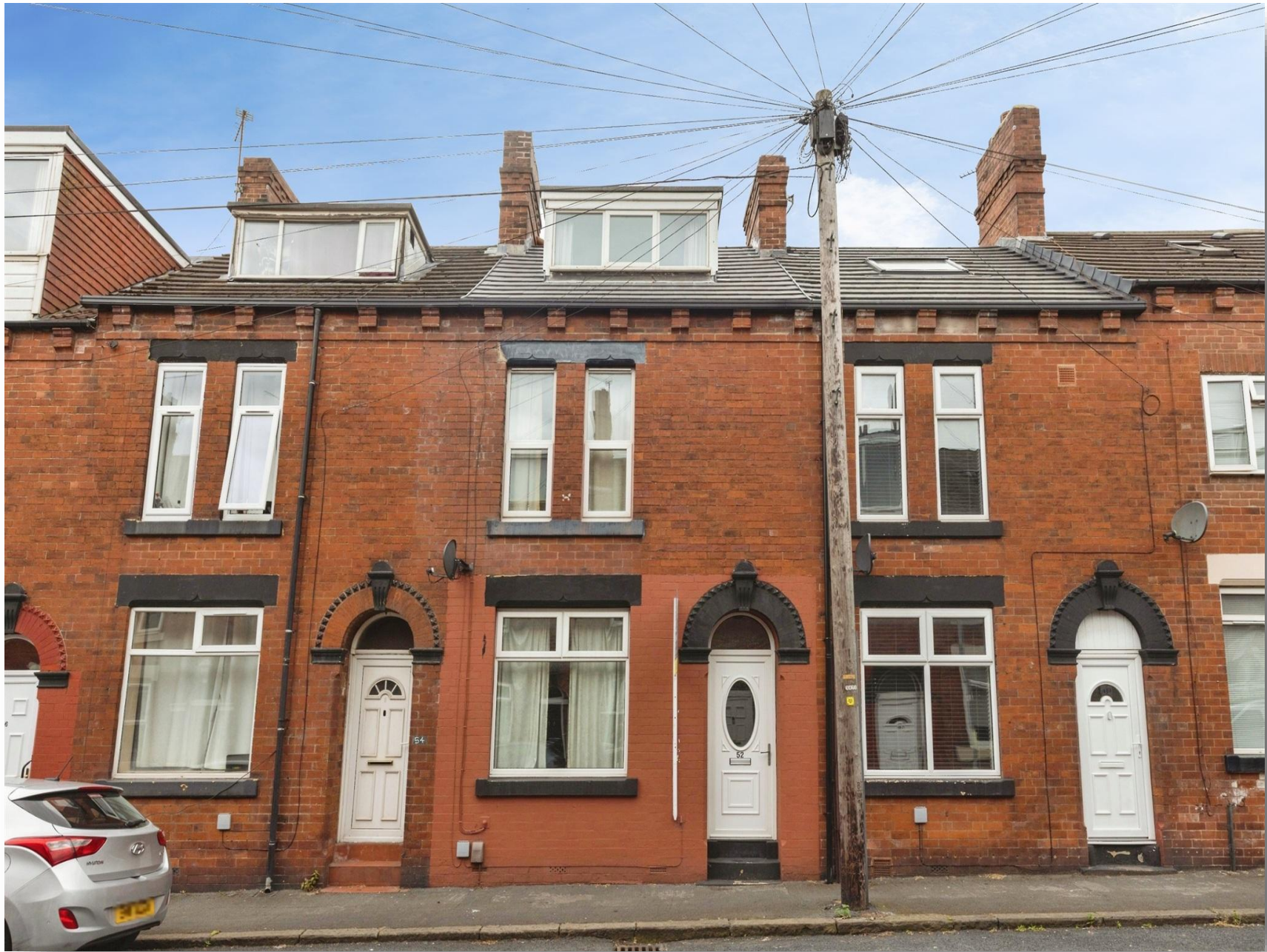
Victoria Grove, Leeds LS9 9DW
