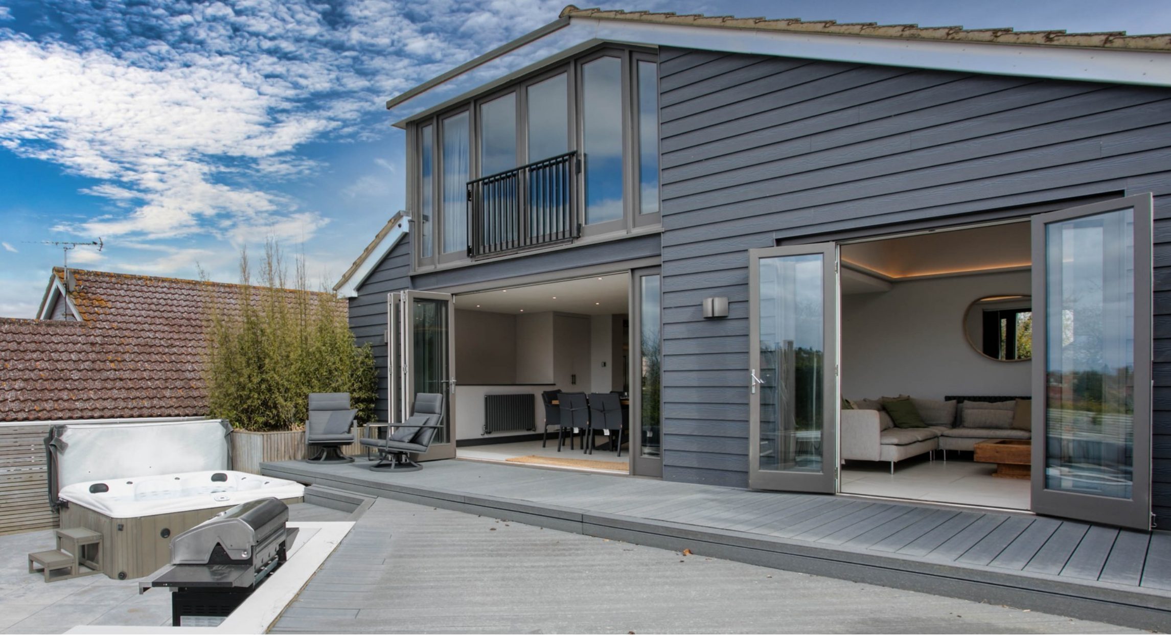
Manorside, Dersingham PE31 6LE
