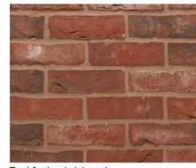
Red facing brickwork
