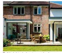
Full height window to rear bedroom
