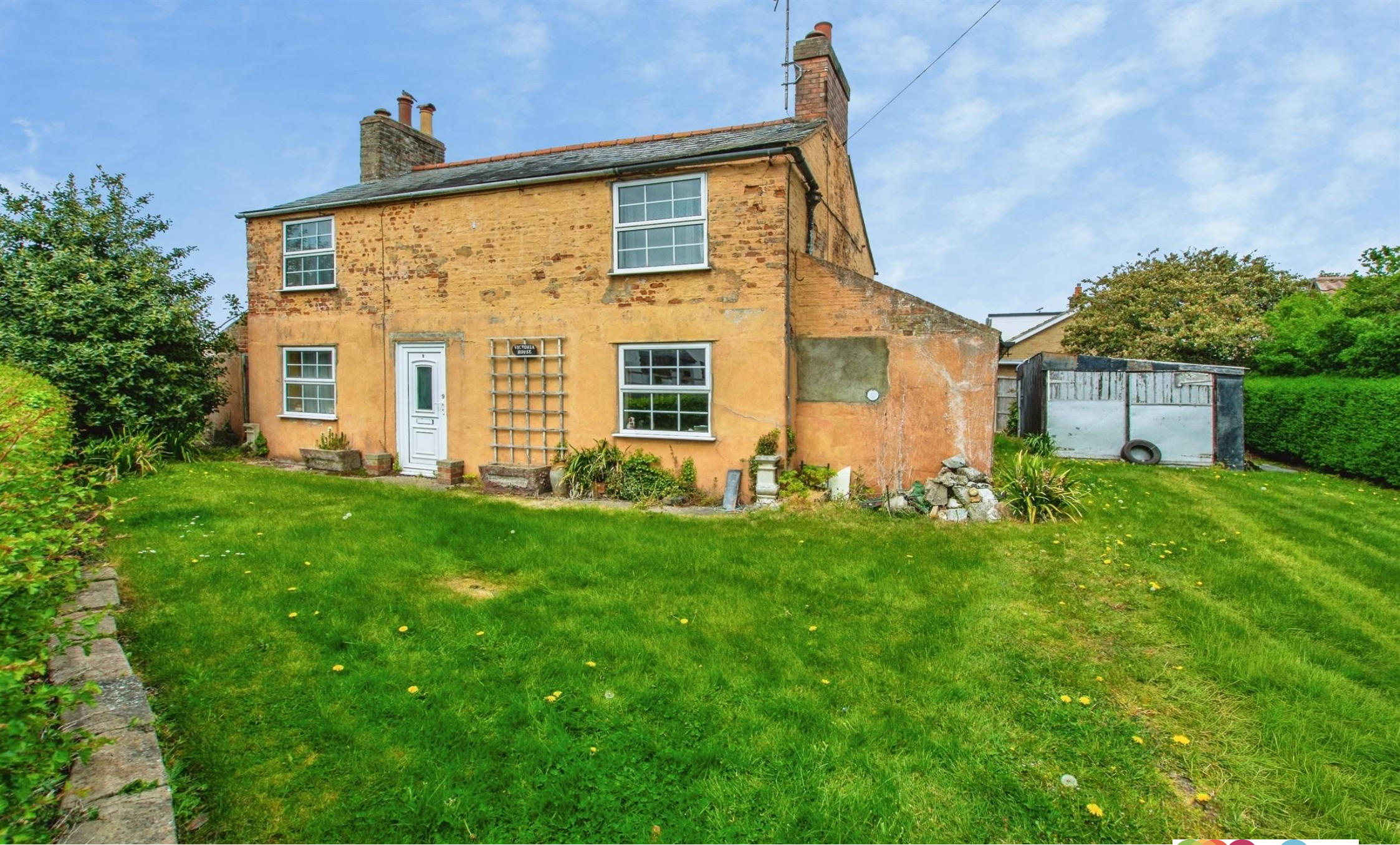
Victoria House School Lane, Lutton Spalding PE12 9HW
