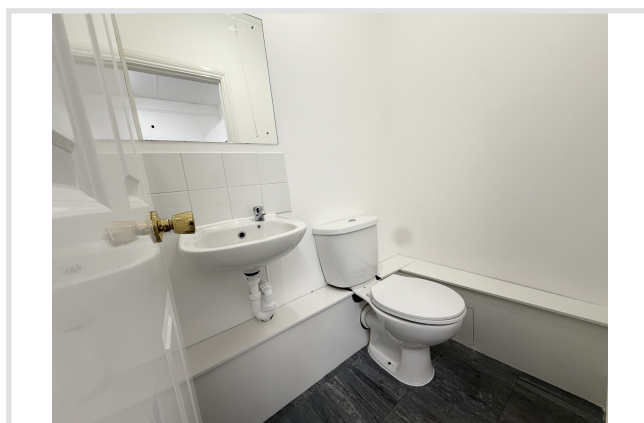
Private WC facilities
