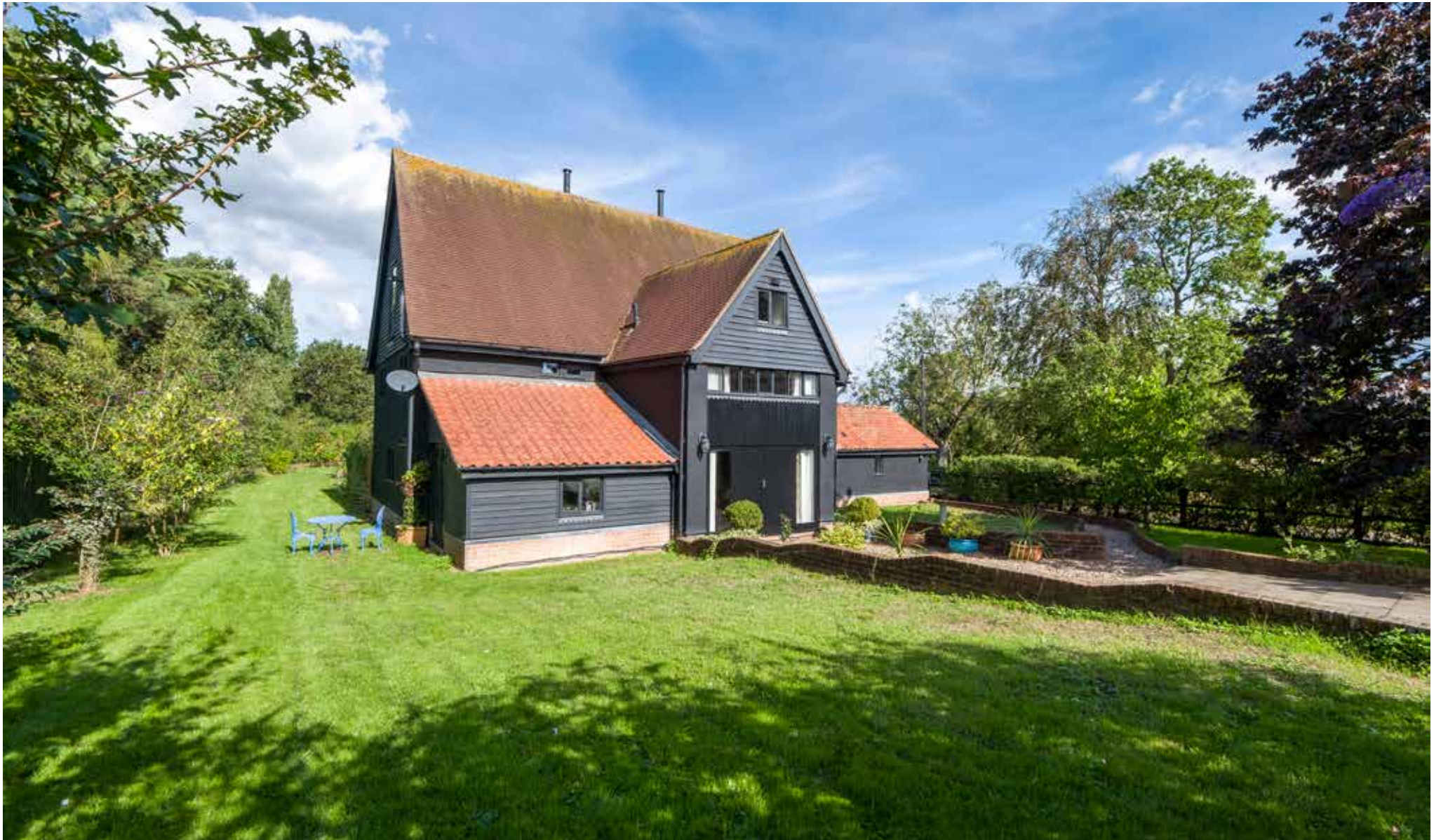
Park Farm Barn Brome Avenue | Eye | Suffolk | IP237HW
