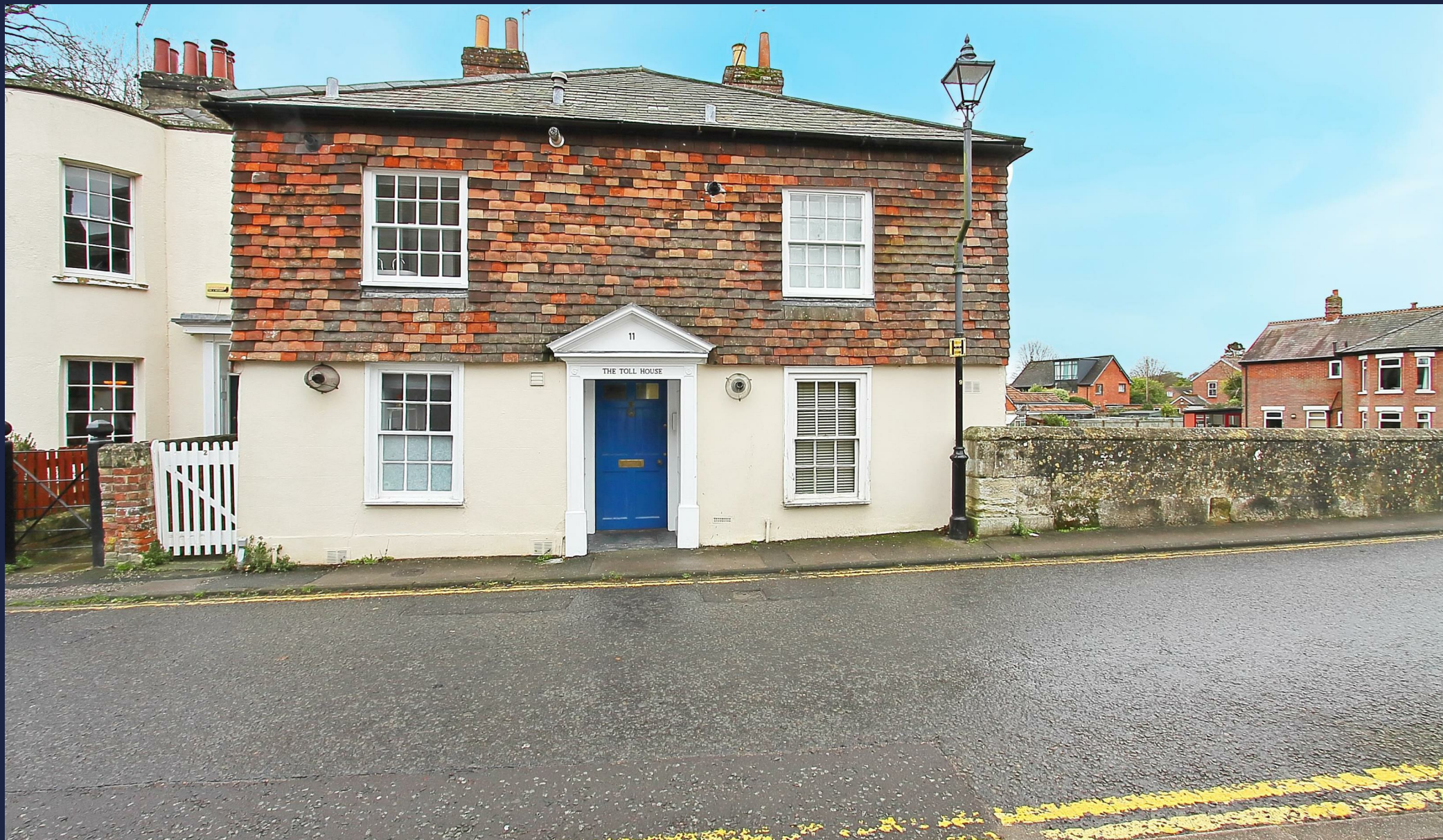
4 The Toll House, 11 St Nicholas Road, Salisbury
