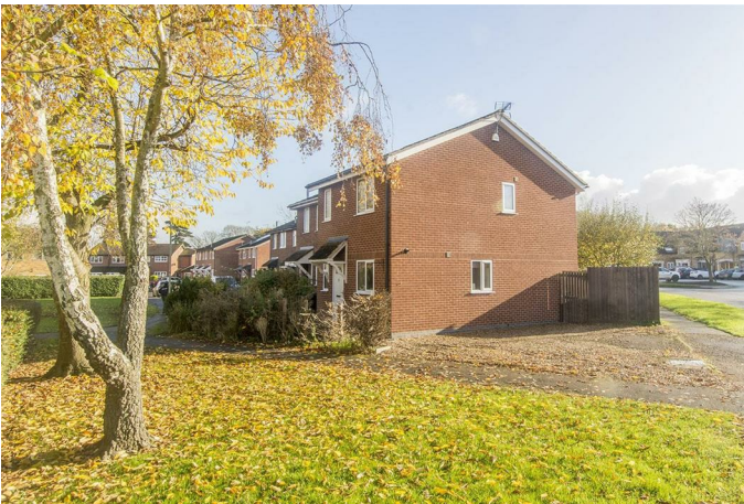
Side Elevation photo
