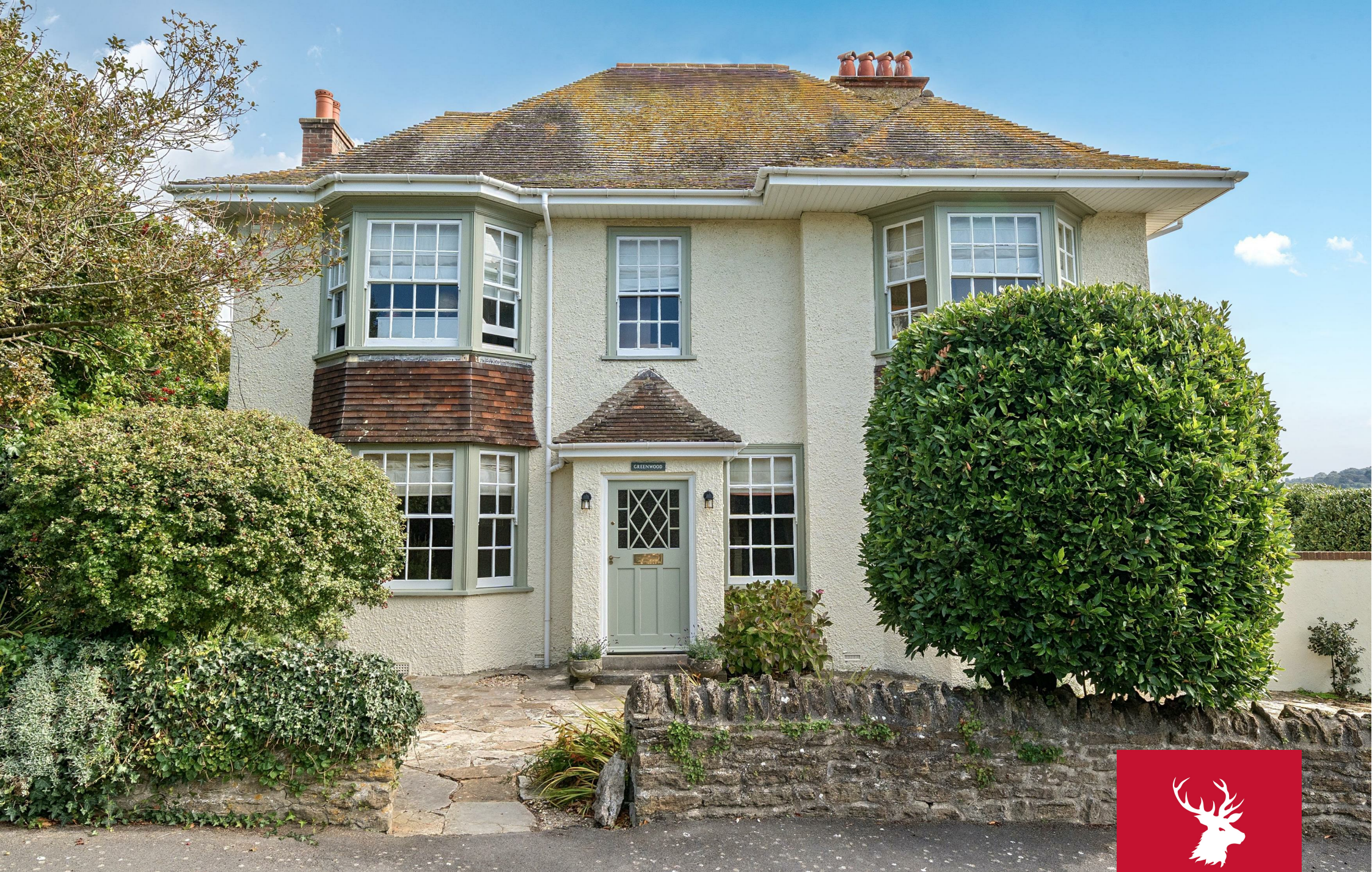
Greenwood, Allington Park
