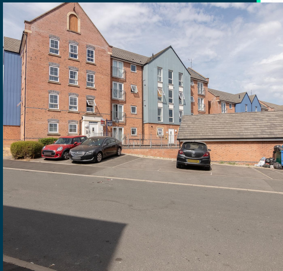
Quayside Court, Coventry, CV1
