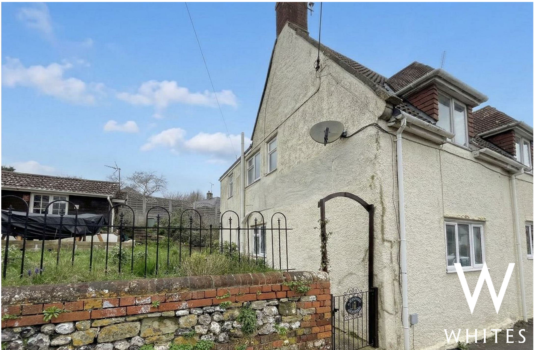
1 Rectory Cottages, South Street, Great Wishford, Salisbury, Wiltshire, SP2
