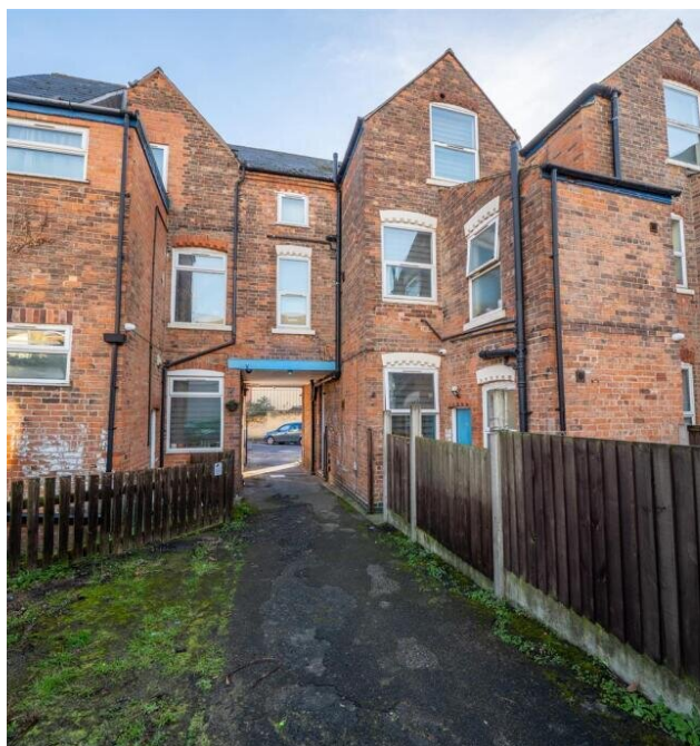
Rear elevations & yards
