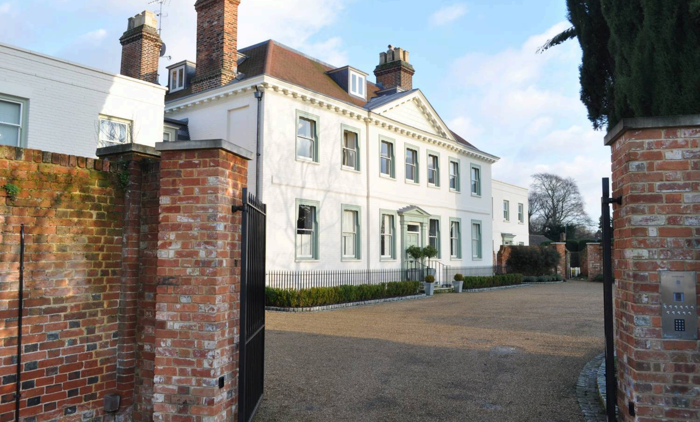
Ashtead Lodge, Parkers Lane Ashtead
