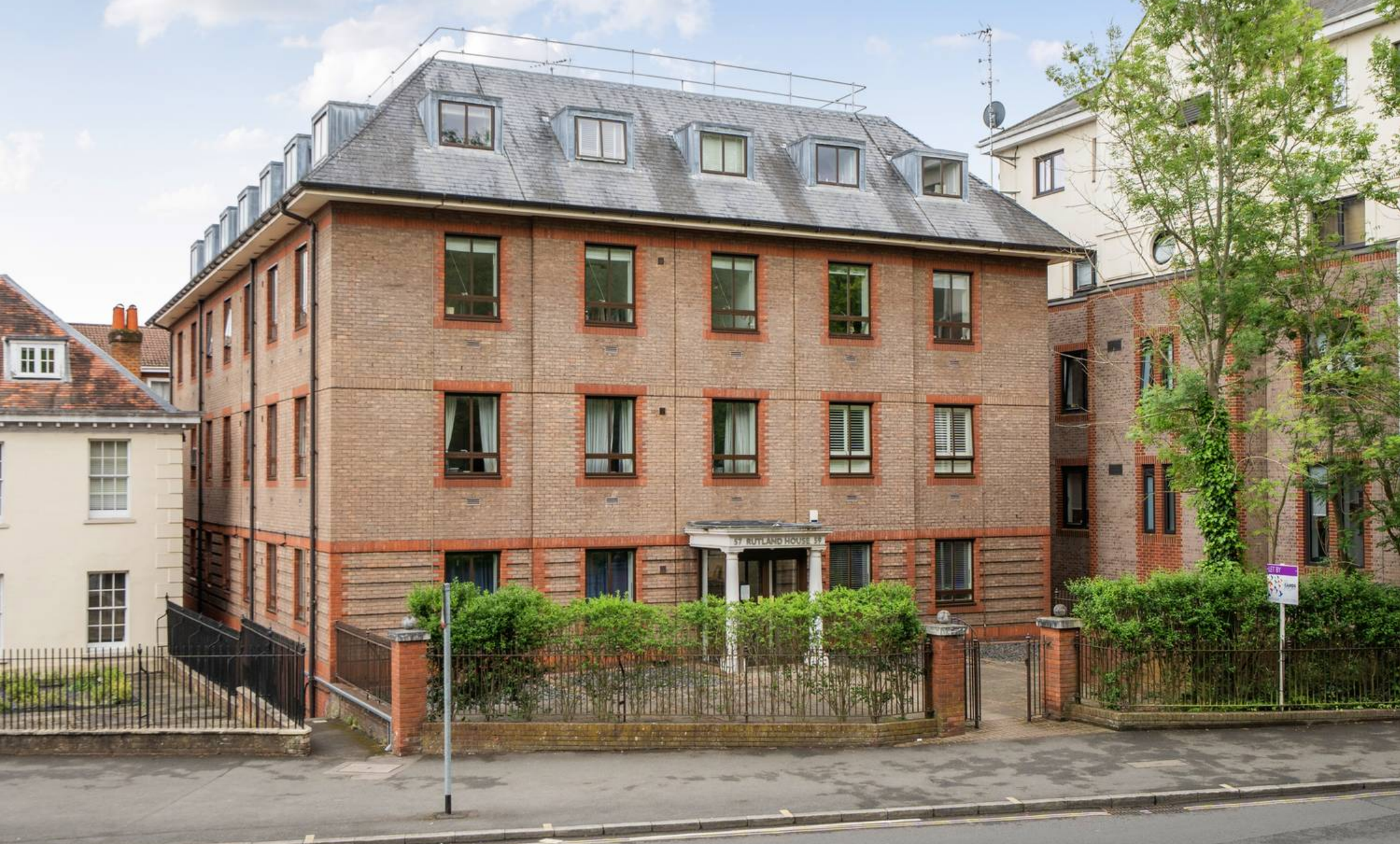
Rutland House, 57-59 South Street, Epsom
