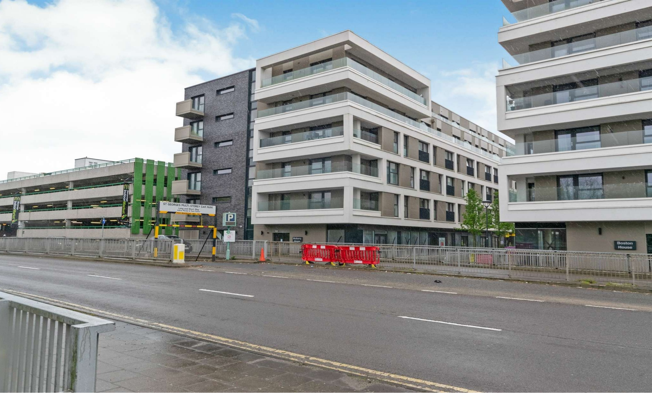
Mulberry House, Park Place, Stevenage, SG1 1BH
