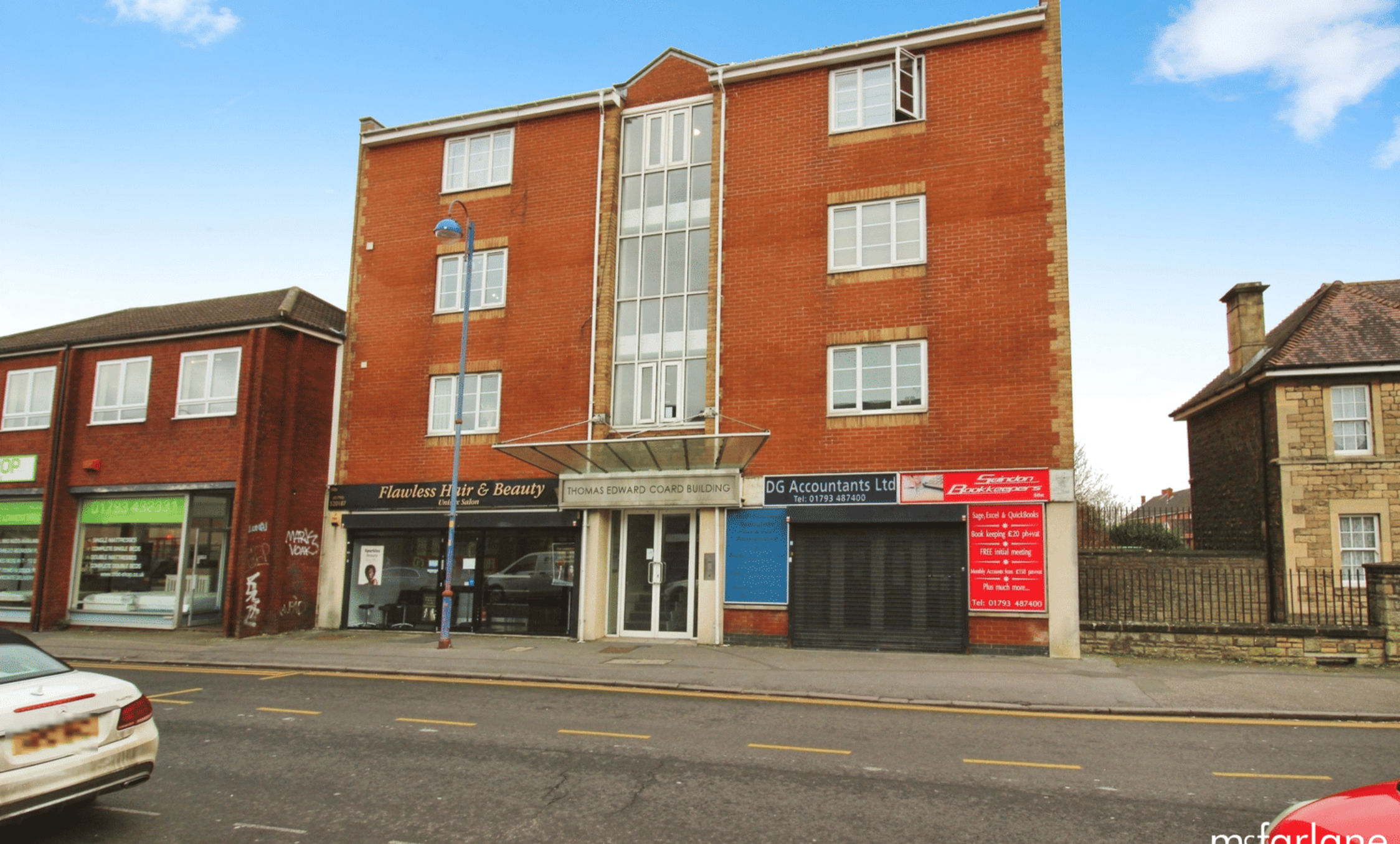
Thomas Edward Coard Building, Cricklade Road, Gorse Hill Swindon
