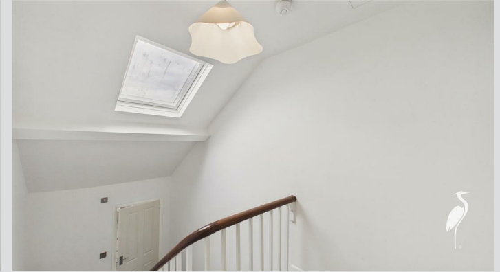
Skylight window and access point to loft.
