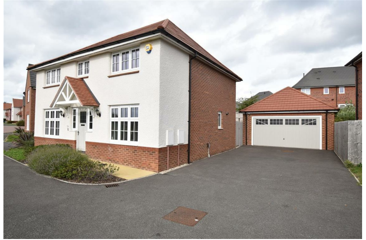
Frontage & Side Driveway
