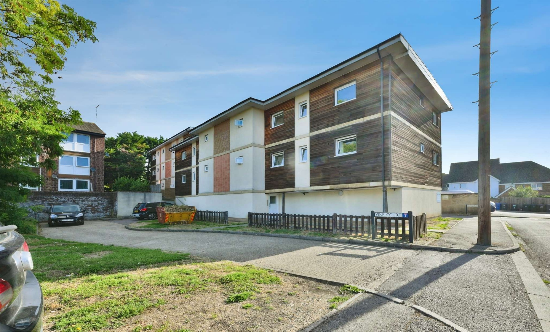
Vine Court, Francis Road, Ware SG12 9GZ
