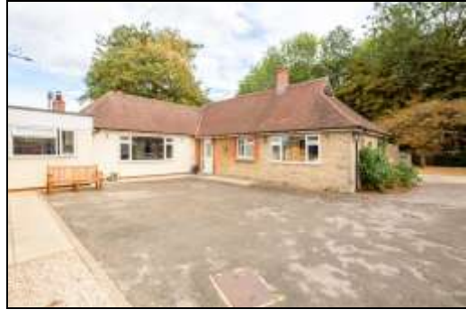
Bungalow Part (Flat roof kitchen connecting the two)
