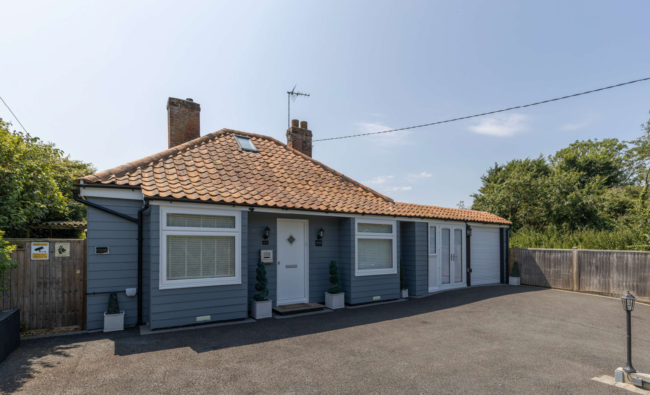
WOOD END RISSEMERE LANE EAST, REYDON
