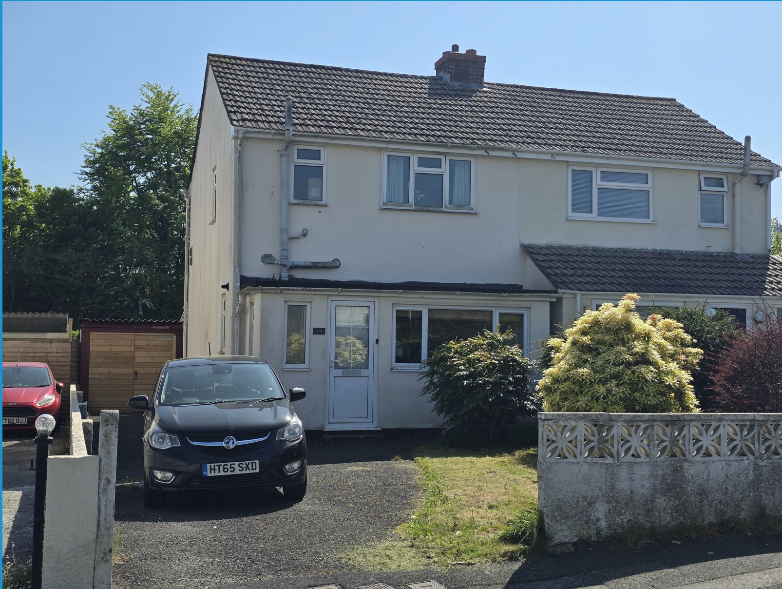
St. Johns Road Launceston | Cornwall
