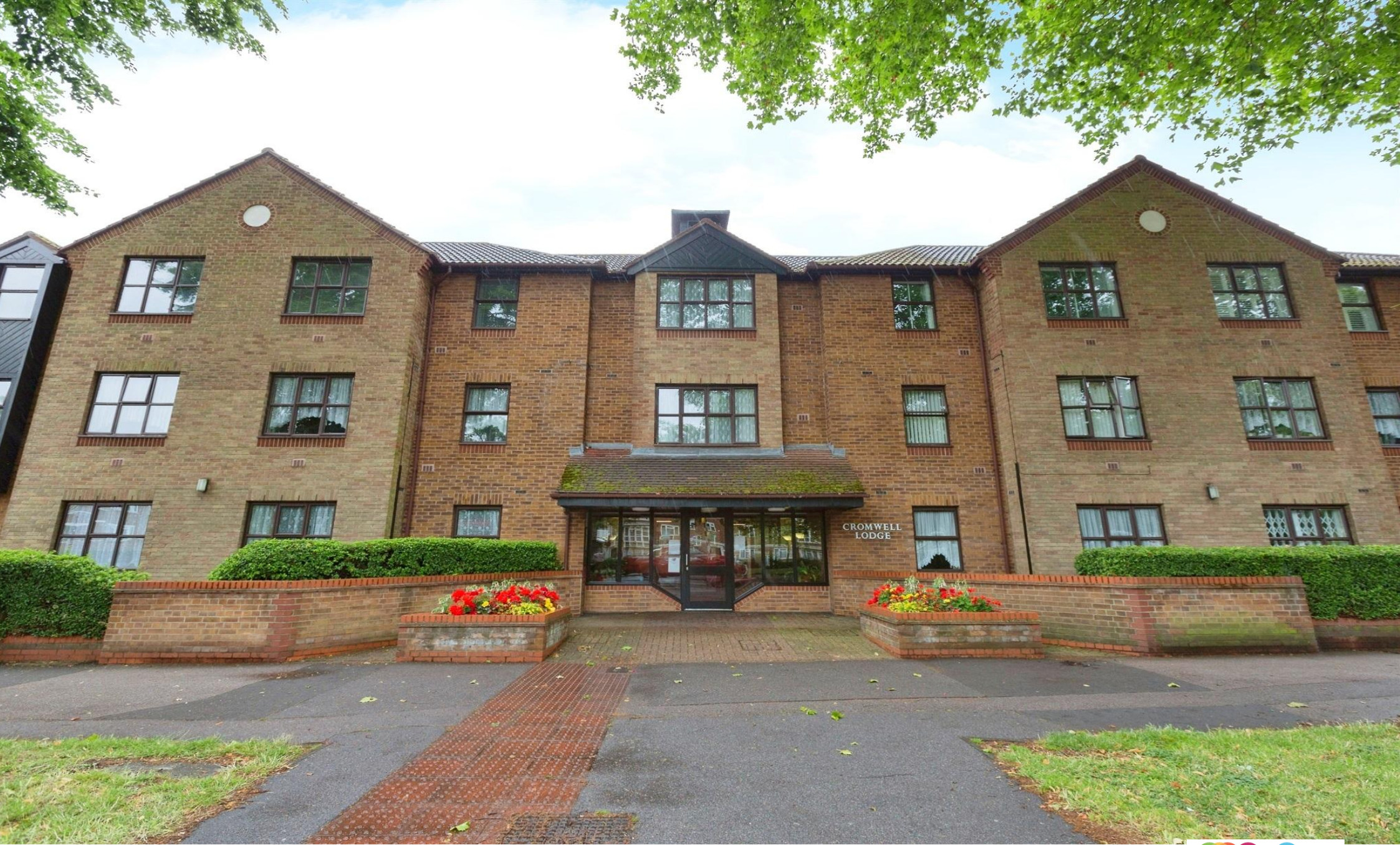
Cromwell Lodge, Longbridge Road, Barking, IG11 8UB
