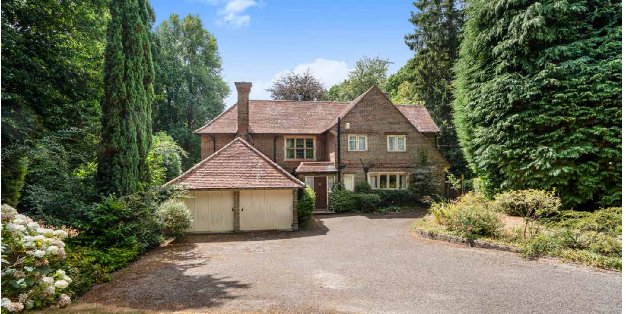
THE GATE HOUSE, MIDHURST ROAD, HASLEMERE
