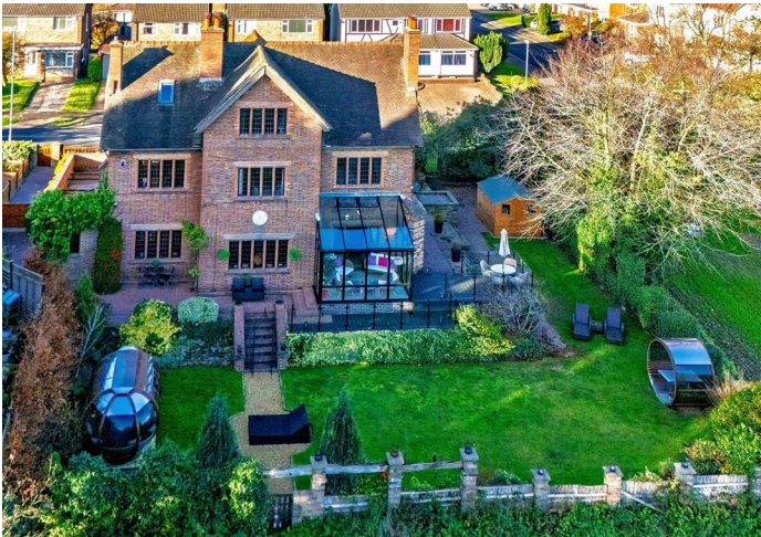
Rear Aerial View
