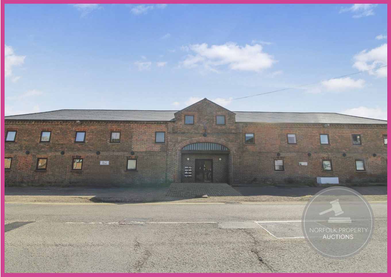
West Bank Sutton Bridge Spalding PE12 9TU
