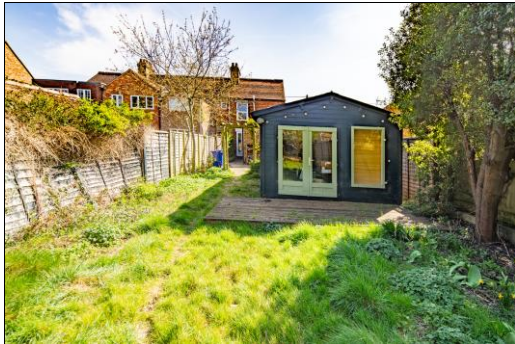
Rear Elevation and Garden Office
