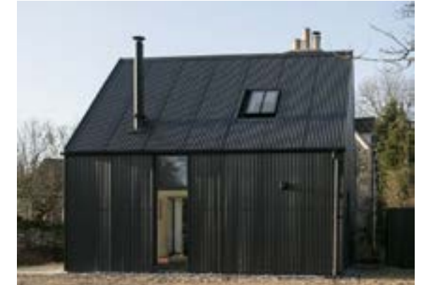
Corrugated metal sheets for roof.
