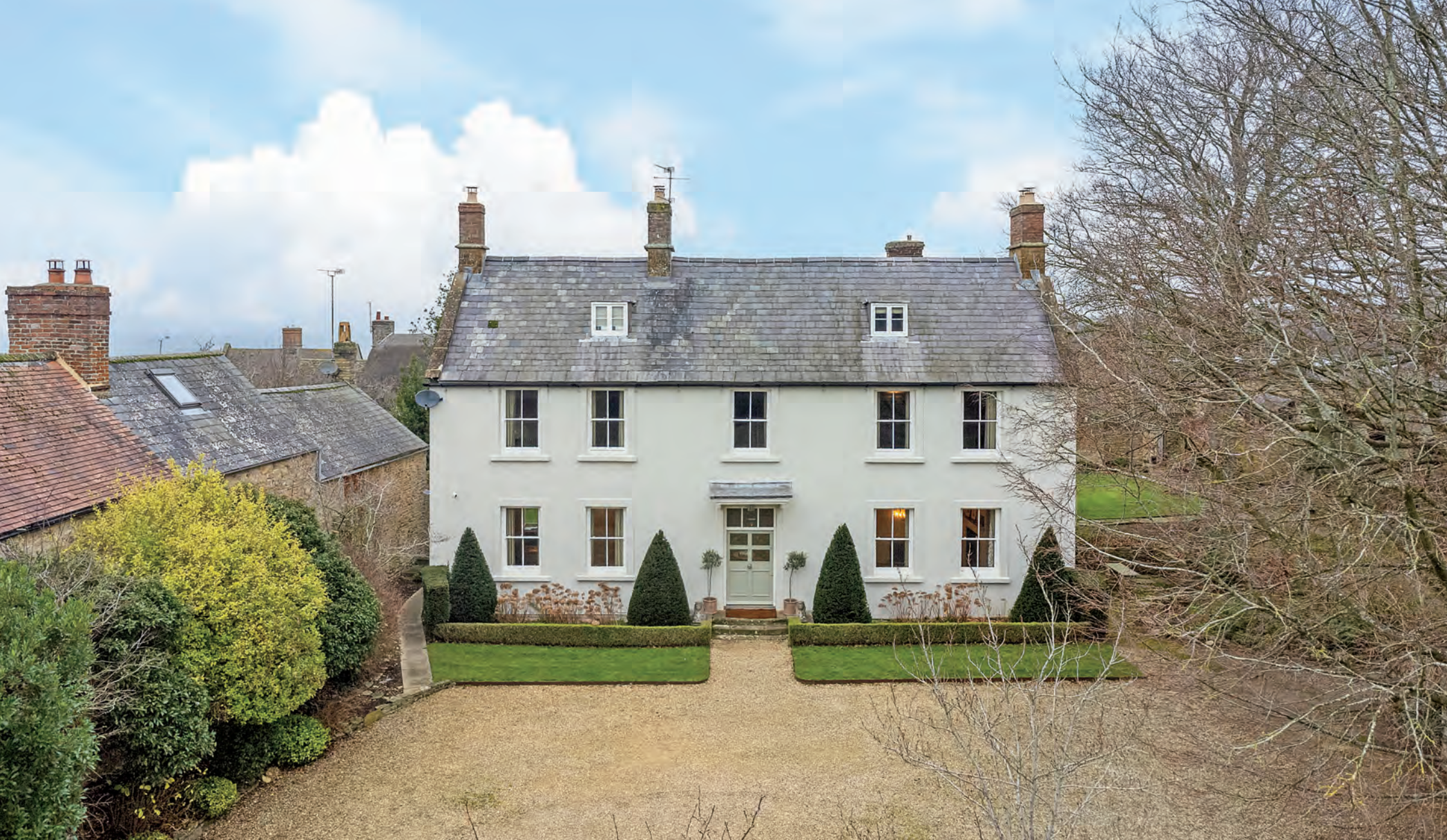
Catton House 10 The Square | Aynho | Banbury | Oxfordshire | OX17 3BL
