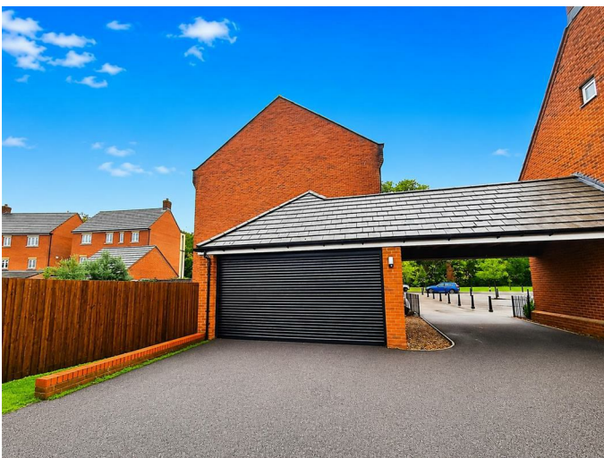
Garage and Driveway
