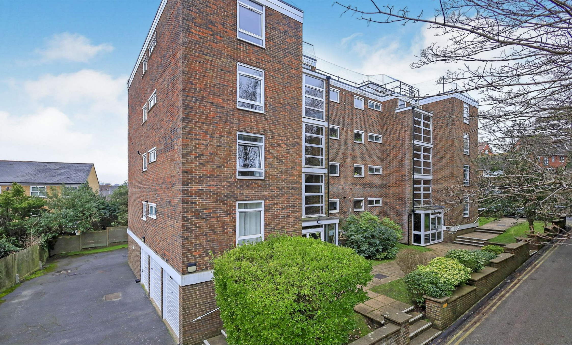
Glenthorne House Arundel Road, Eastbourne BN21 2EZ
