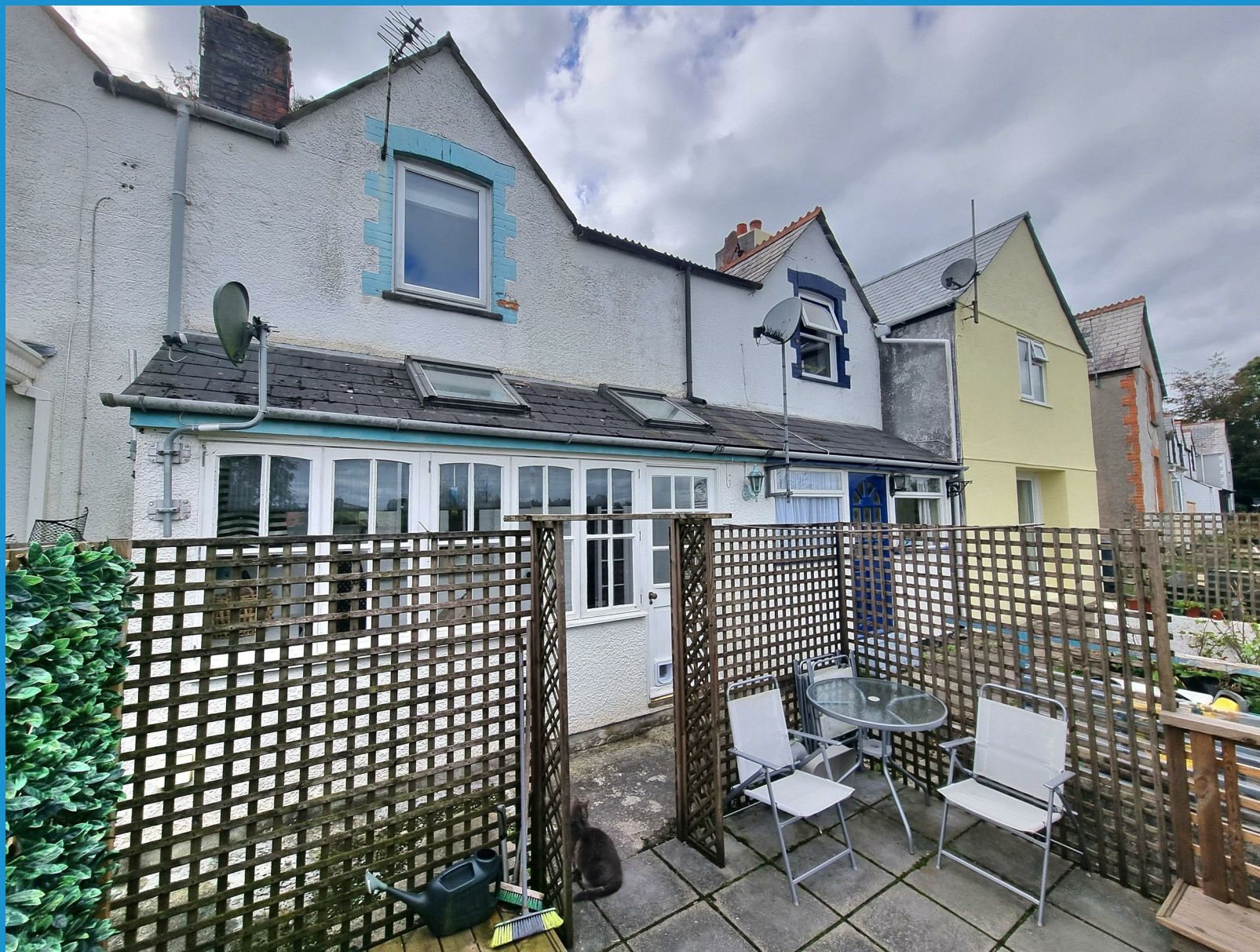
11 Hillpark Cottages Launceston | Cornwall
