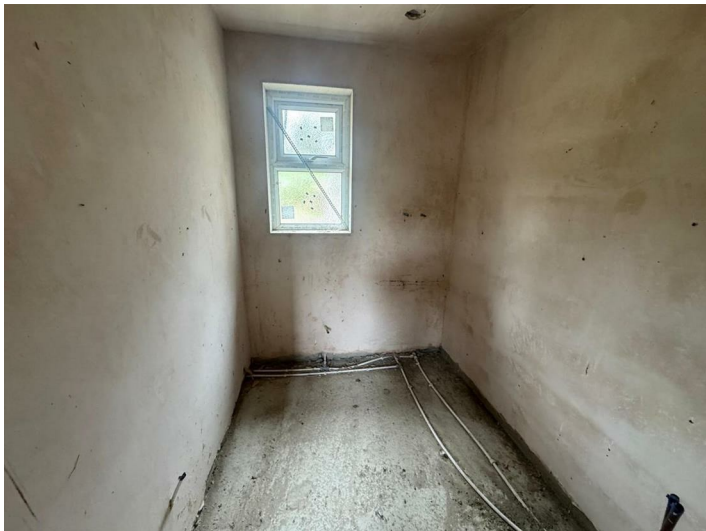
SHOWER ROOM (possible) 6'6 x 5'5 (1.98m x 1.65m )
