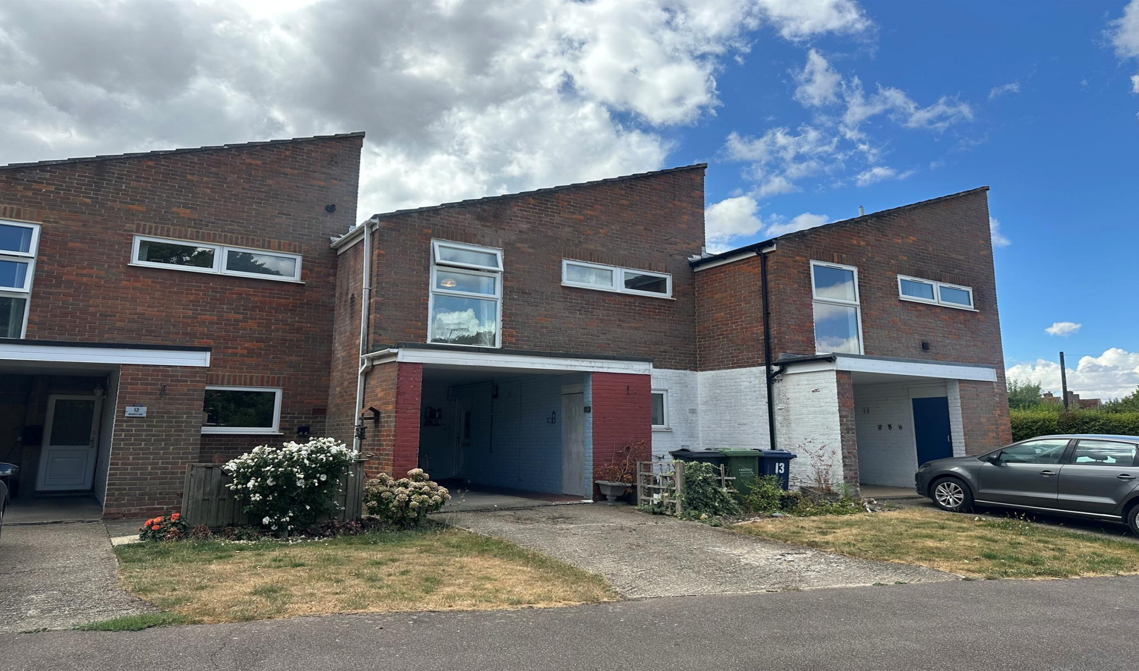
Meades Lane, Chesham HP5 1ND
