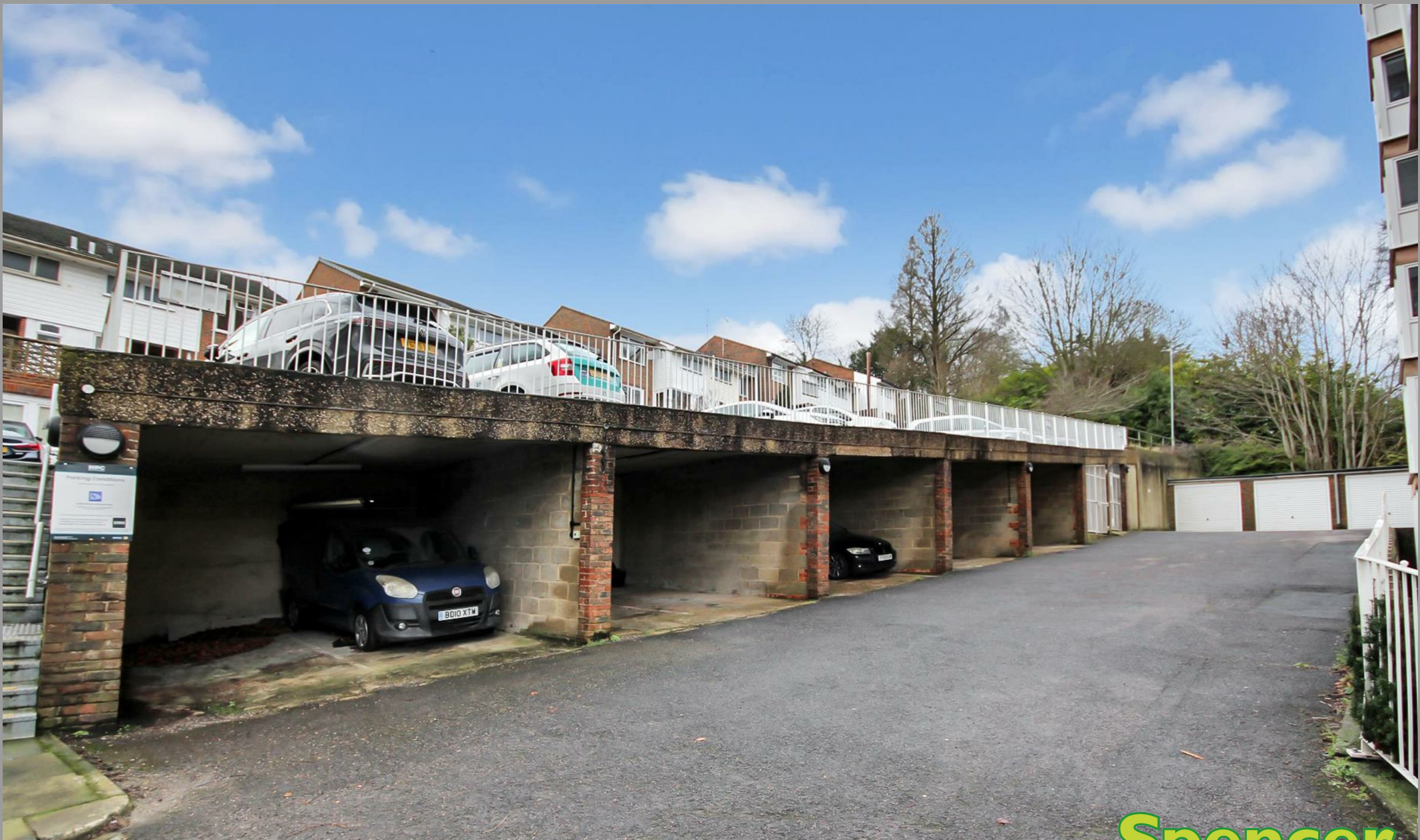
Carport 12, Preston Grange, Brighton, BN1 6BH
