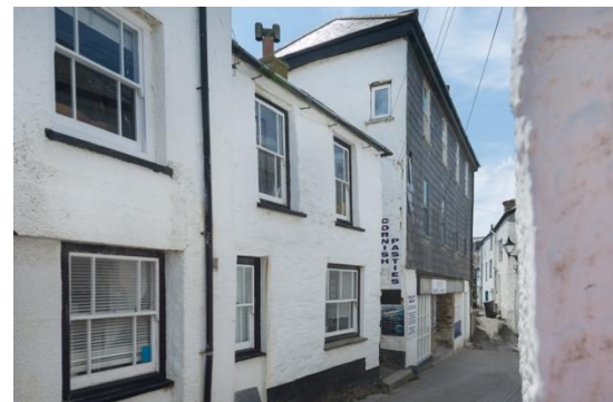
External of Stanley House with its slate hung façade
