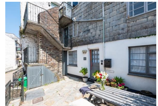
External staircase from The Old Bakehouse
