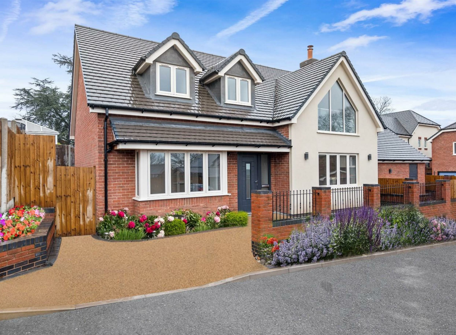
Pumphouse Lane, Redditch
