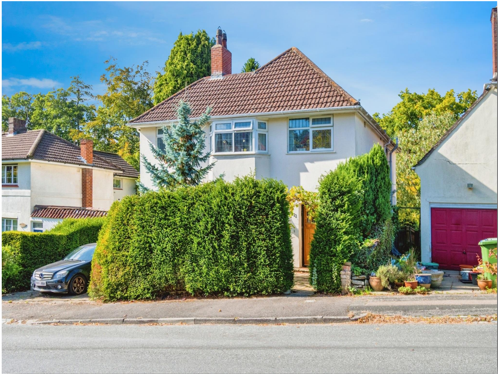
Bassett Dale, Southampton SO16 7GT
