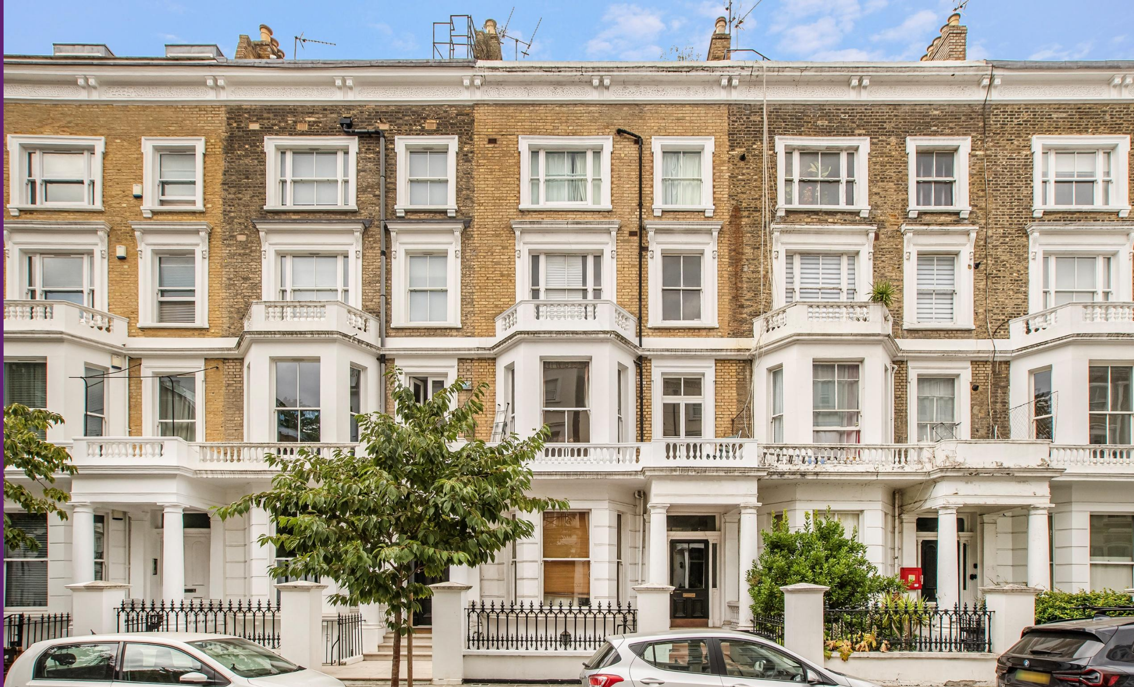
Lexham Gardens Kensington, W8
