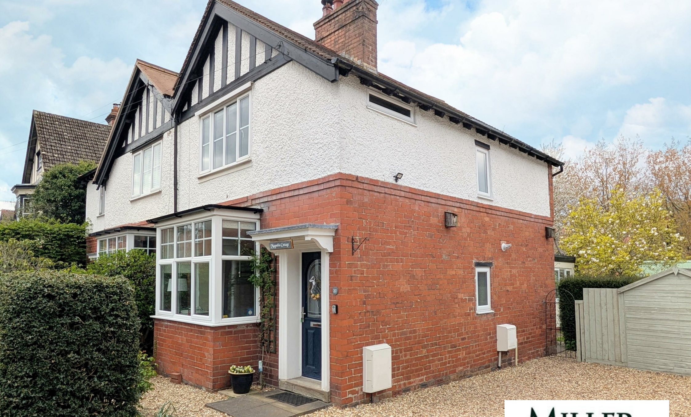
Magnolia Cottage, 50 Watling Street South, Church Stretton, SY6 7BQ
