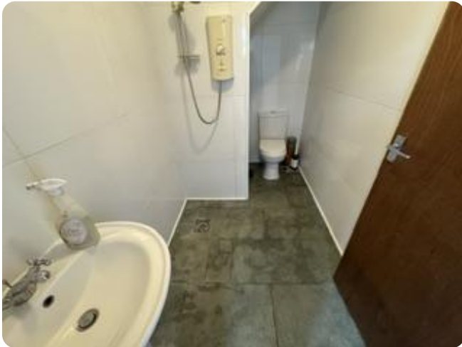
BATHROOM TWO — GROUND FLOOR
