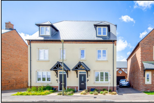
Front, Garage & Driveway for 3 cars
