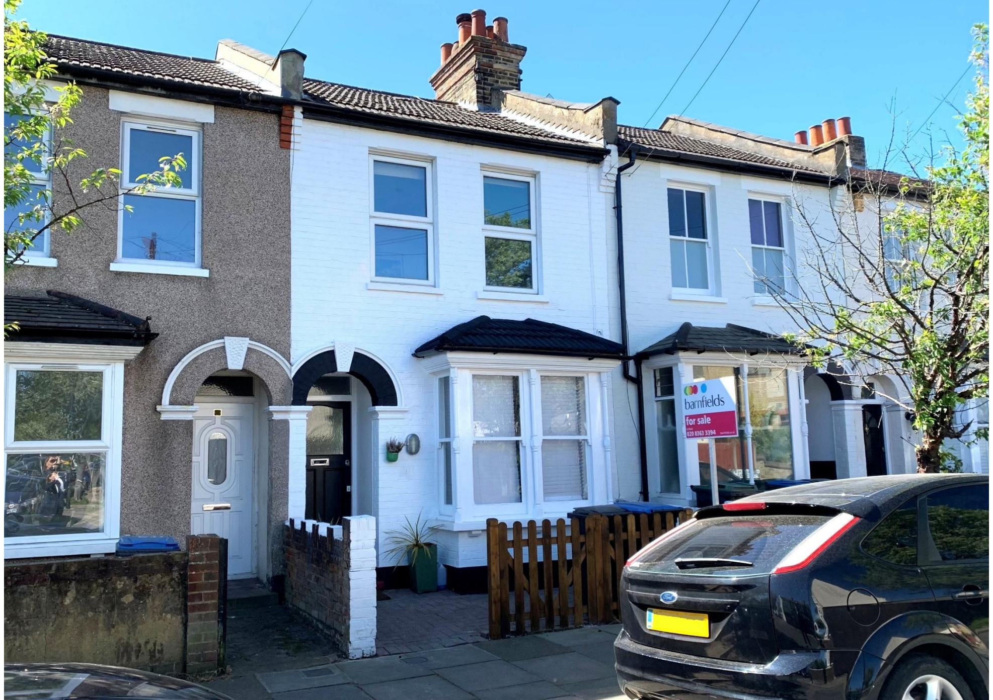
Cross Road, Enfield, EN1 1PD
