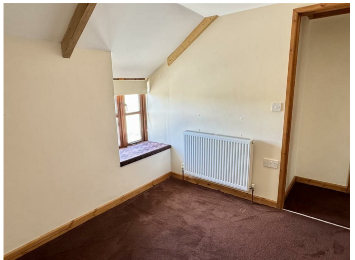
Wood frame double glazed window to side elevation.
