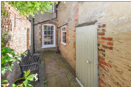
Rear Yard and Shed
