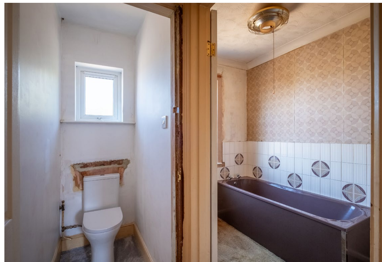
Bathroom and separate WC
