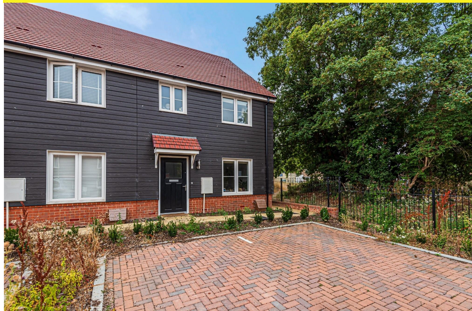
Weave Crescent, Andover
