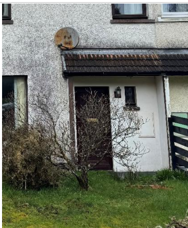
Photo 11 – Canopy roof structure
