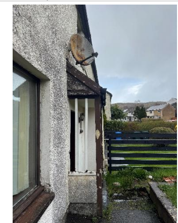
Photo 6 – Front entrance canopy structure
