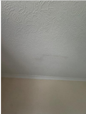
Photo 18 – location of discolouration on living room ceiling
