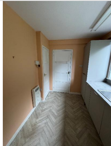
Photo 21 – Kitchen in good condition
