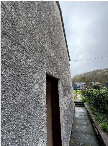
Photo 15 – Condition of gable end
