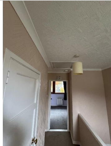
Photo 25 – First floor hallway and attic hatch
