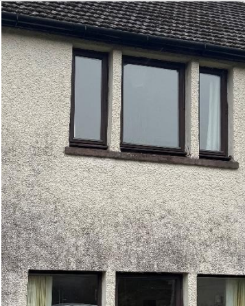
Photo 3 – Cracking noted at base of first floor bedroom window piers on front elevation
