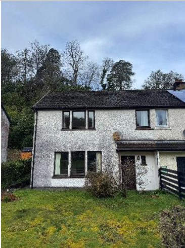
Photo 13 – Roof profile on front elevation
