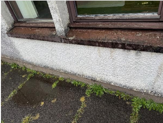
Photo 3 – Cracking noted at base of first floor bedroom window piers on front elevation
