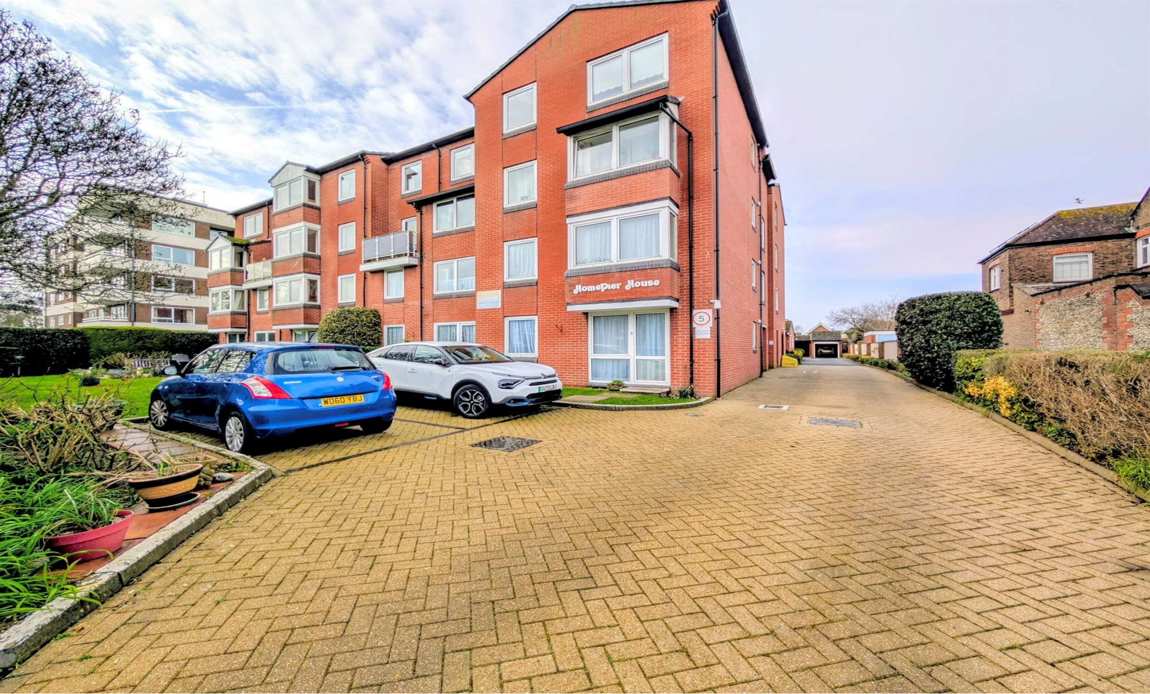
Homepier House Heene Road, Worthing BN11 4PP
