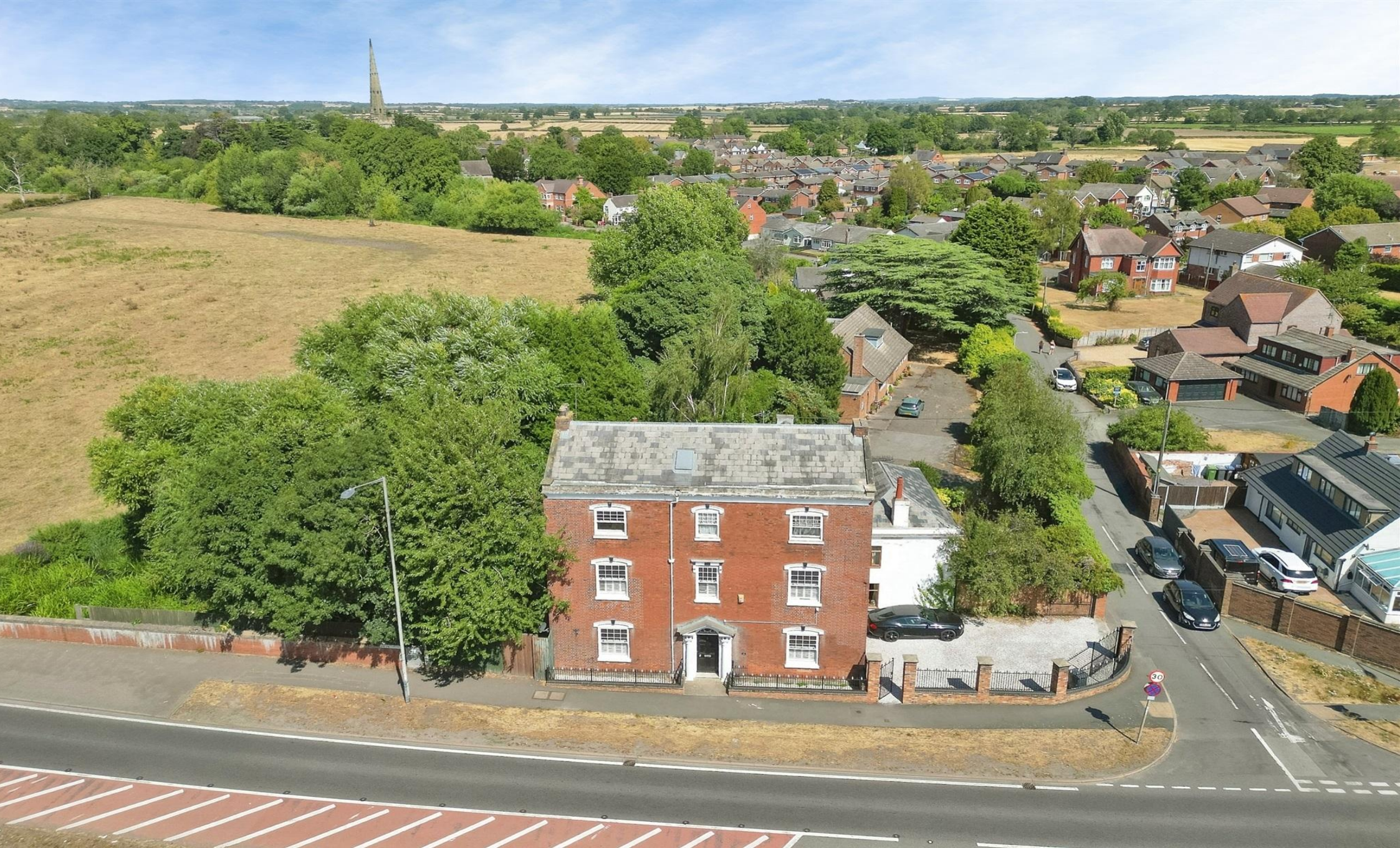
Bridge House, Watling Street, Witherley, Atherstone
